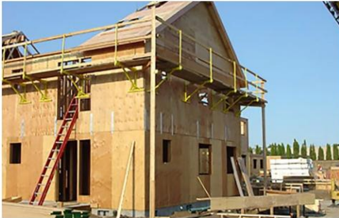
Manufactured exterior carpenter's bracket scaffolding.
