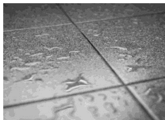
Walking & working surfaces
