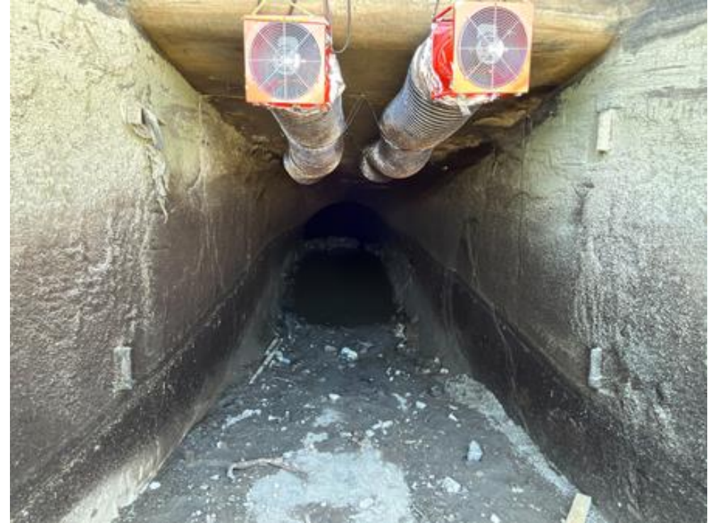
Two 5,500 cfm fans pulling air out of the Siphon Inlet
