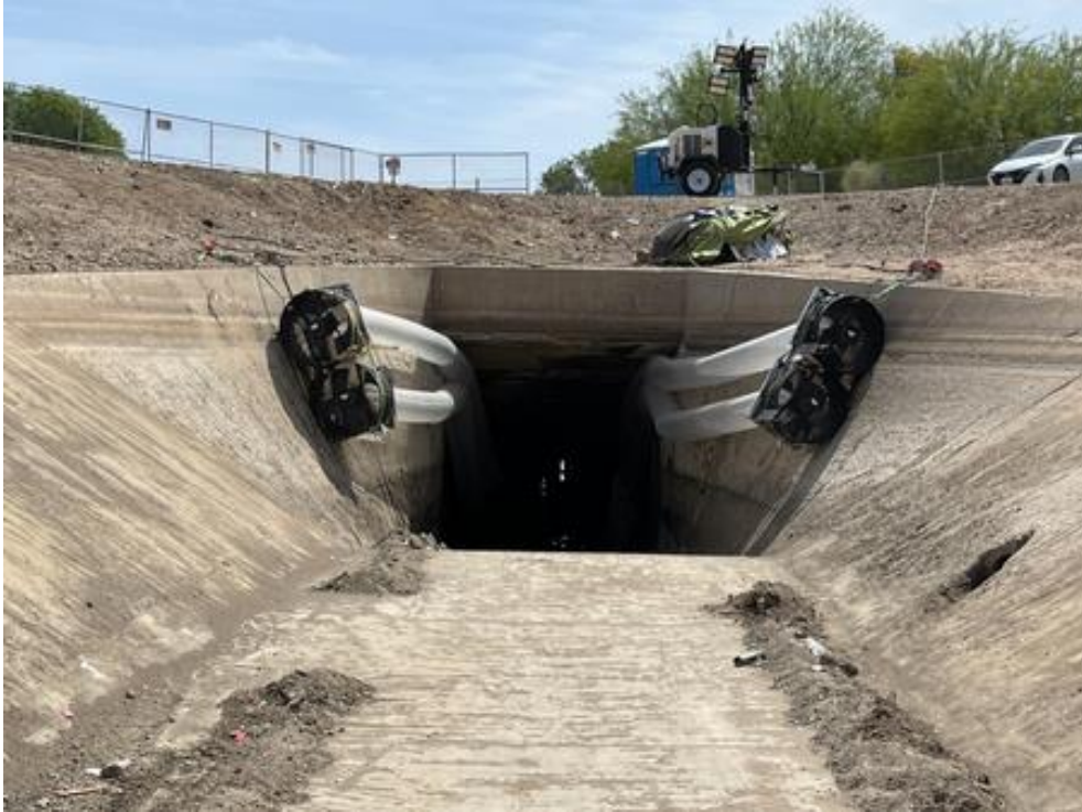
Four 7,800 cfm fans pushing air into the Siphon Outlet
