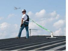
Fall Restraint reduces the likelihood of a fall while fall arrest reduces the severity
