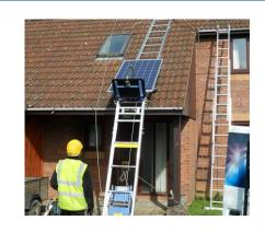
Prevents the activity of lifting solar while hanging over the roof
