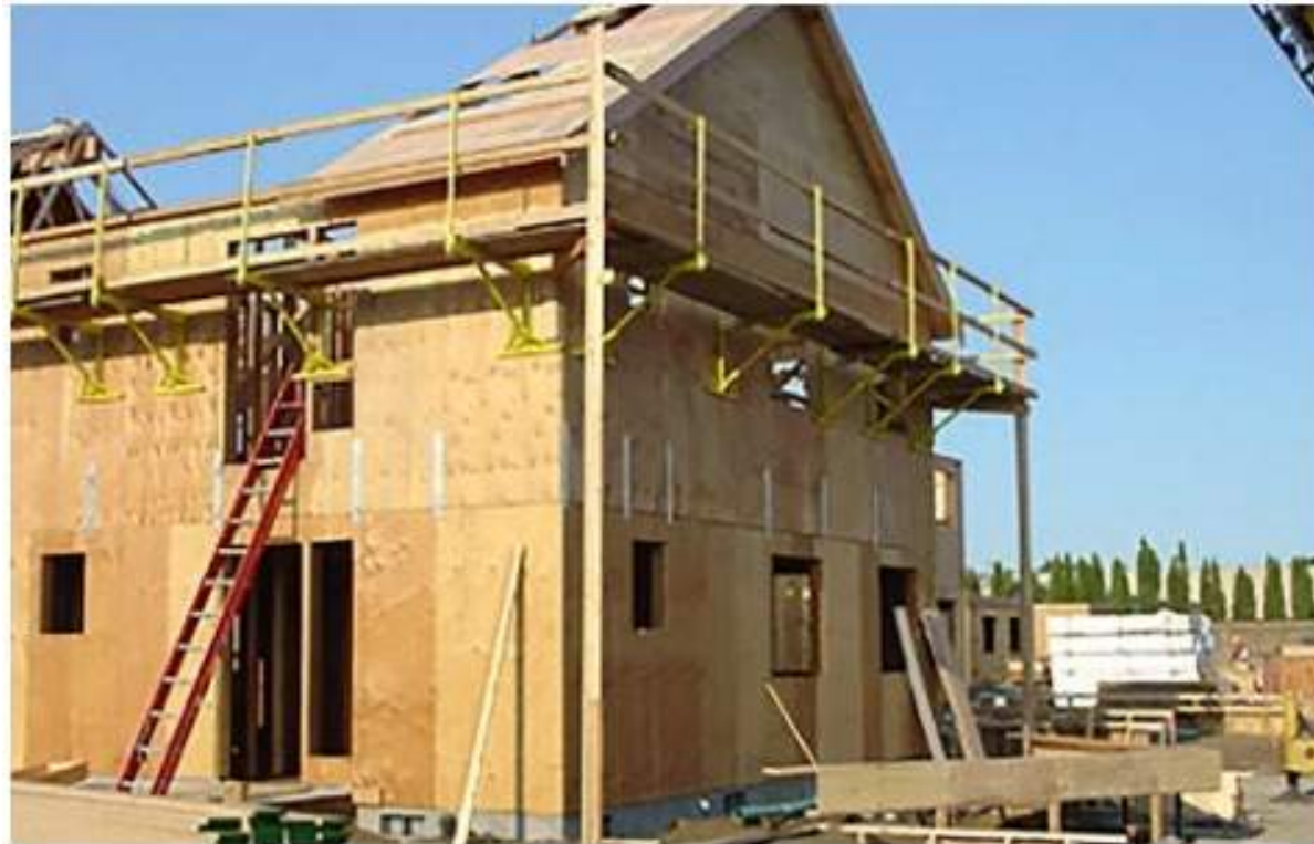
Manufactured exterior carpenter's bracket scaffolding.
